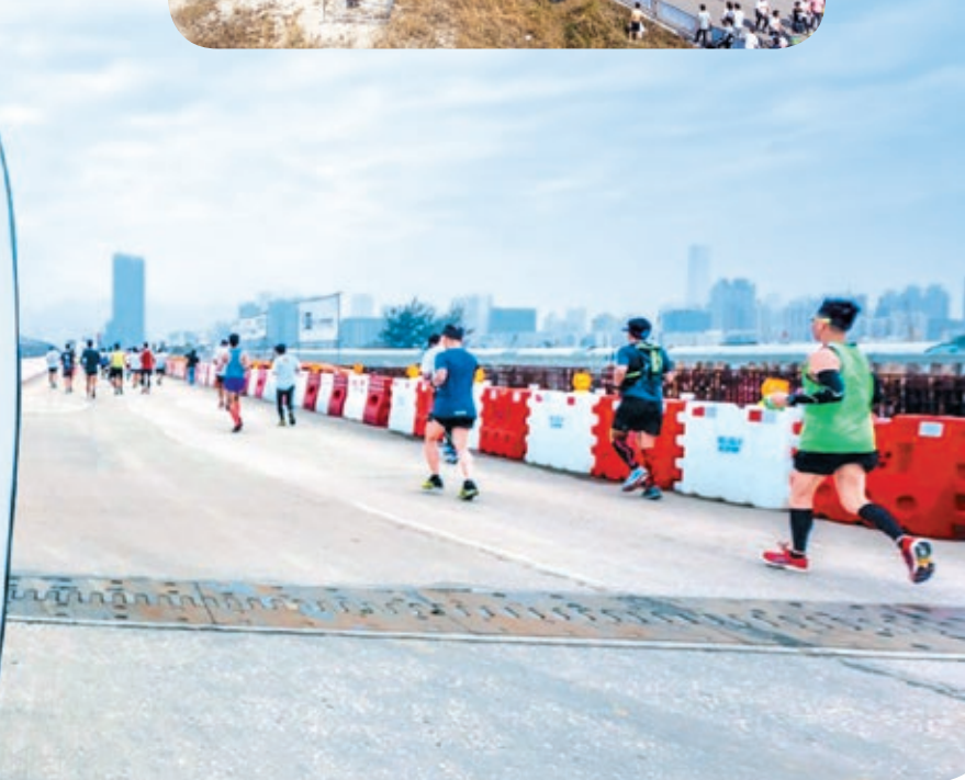
位於前跑道的工地通道首次開放 A construction access at the former runway was opened for the first time
